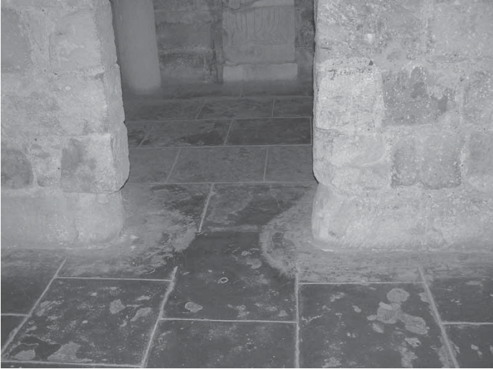
Fig. 29: Limassol Castle, lower level of cells, detail of transition between fire-damaged original masonry (lowest ashlar course on the left, two lowest courses on the right) and later restoration [M. Olympios].
